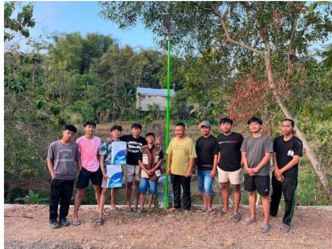
Picture 3. Installation of solar panel lights on posts at designated road locations
